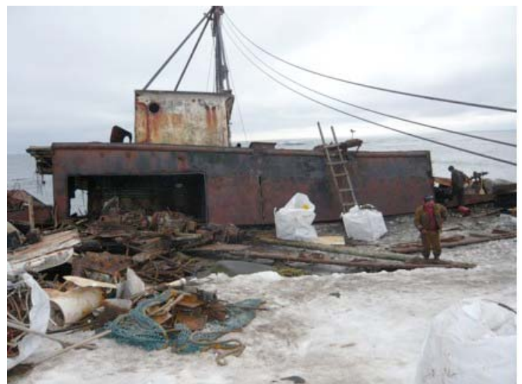
(Above) The Ocean Clipper ran aground on a vital Northern Fur Seal rookery on St. Paul Island, Alaska (Below) Working in sub-freezing temperatures, the ship was carefully cut apart and hauled piece by piece off the rookery using an aerial cable system.
